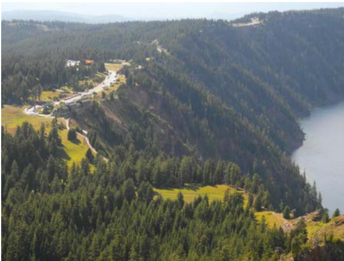
Figure 8. Crater Lake Lodge. Slope movements are apparent on the caldera wall below Crater Lake Lodge, where the historic lodge is located less than 15 m (50 ft) from the rim. The caldera wall slopes very steeply for about 270 m (900 ft) down to Crater Lake. The lodge was constructed on top of a thick, unconsolidated deposit of dacite of Munson Valley (PEd vb ), which consists of material transported by hot debris avalanches derived from the collapse of an unstable lava dome high on Mount Mazama about 35,000 years ago. National Park Service photograph.
