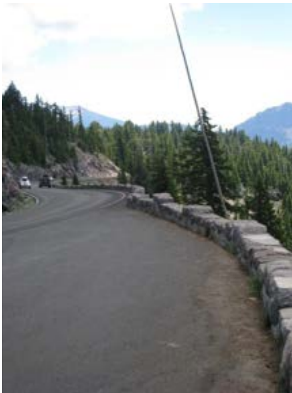
Buildings and Structures #2: Curvilinear stone masonry guard wall at Union Peak substation (Gjesfjeld, PWR, 2010).
