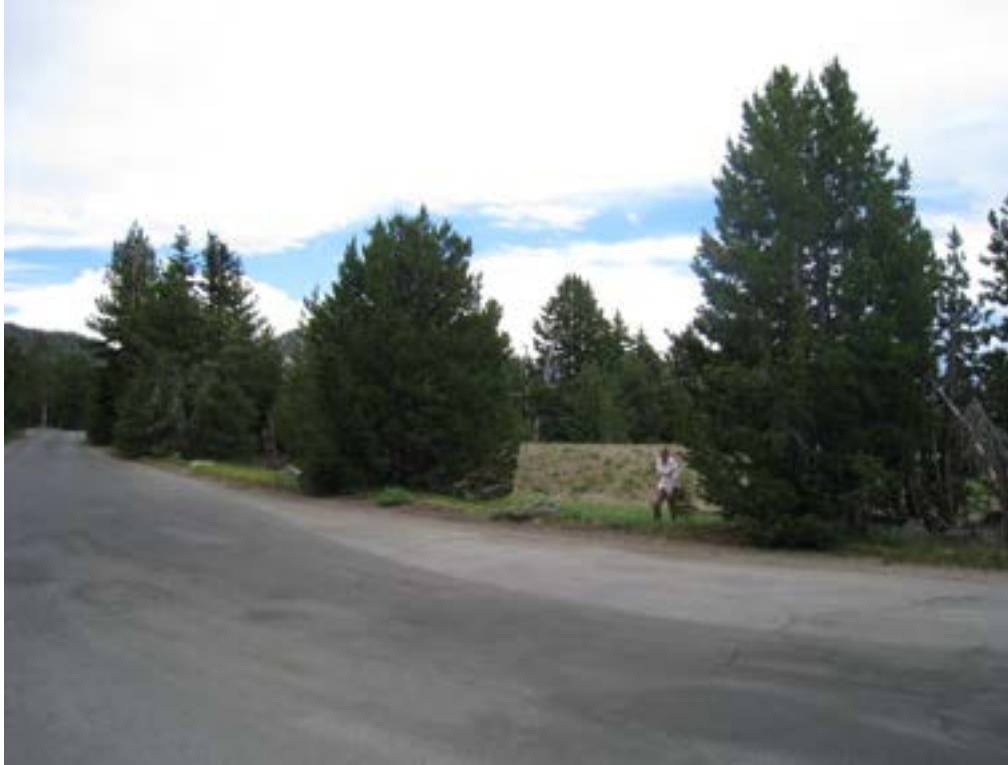
Vegetation #3: Island of vegetation separating Rim Drive from the Sentinel Rock (Victor View) substation (Gjesfjeld, PWR, 2010).
