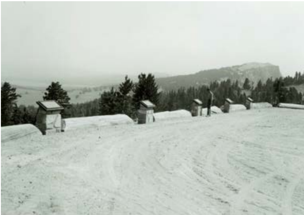
History # 10: The Diamond Lake substation with wayside exhibits located between log guardrails, 1959 (CLNPMAC).
