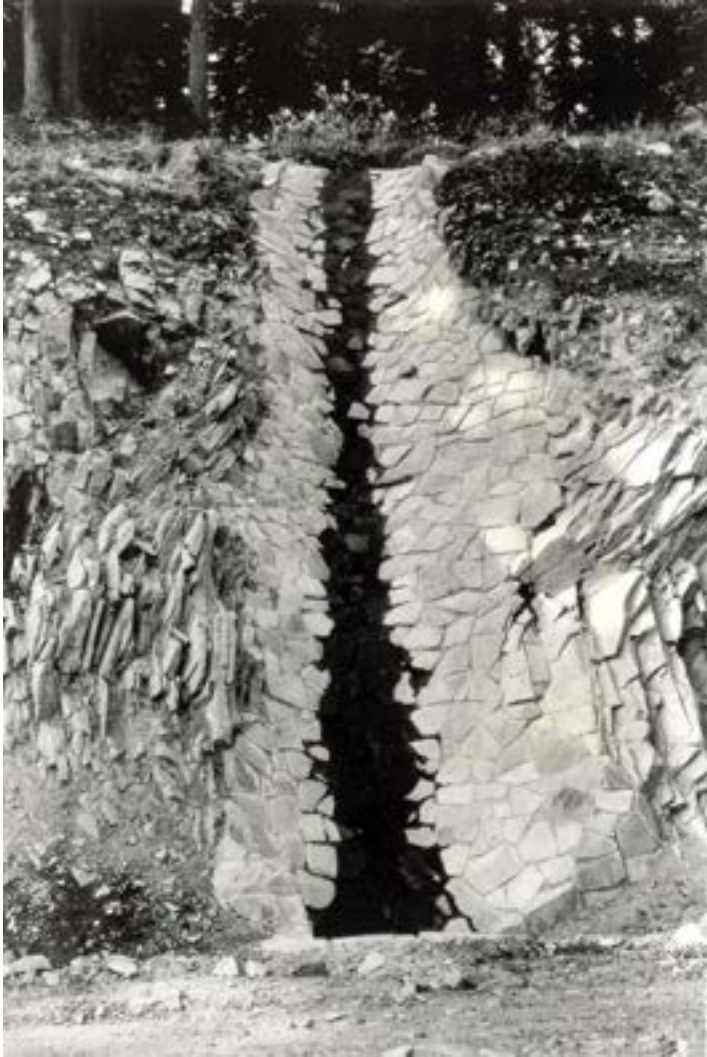
History #8: Stone masonry spillway located along segment 7-D2 (Lange, NARA, RG 79, SB).
