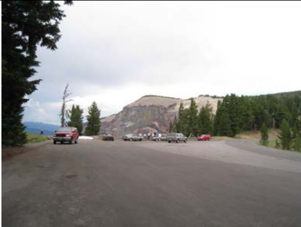
Circulation #13: View of Pumice Castle (Cottage Rocks) substation (Germano, PWR, 2010).
