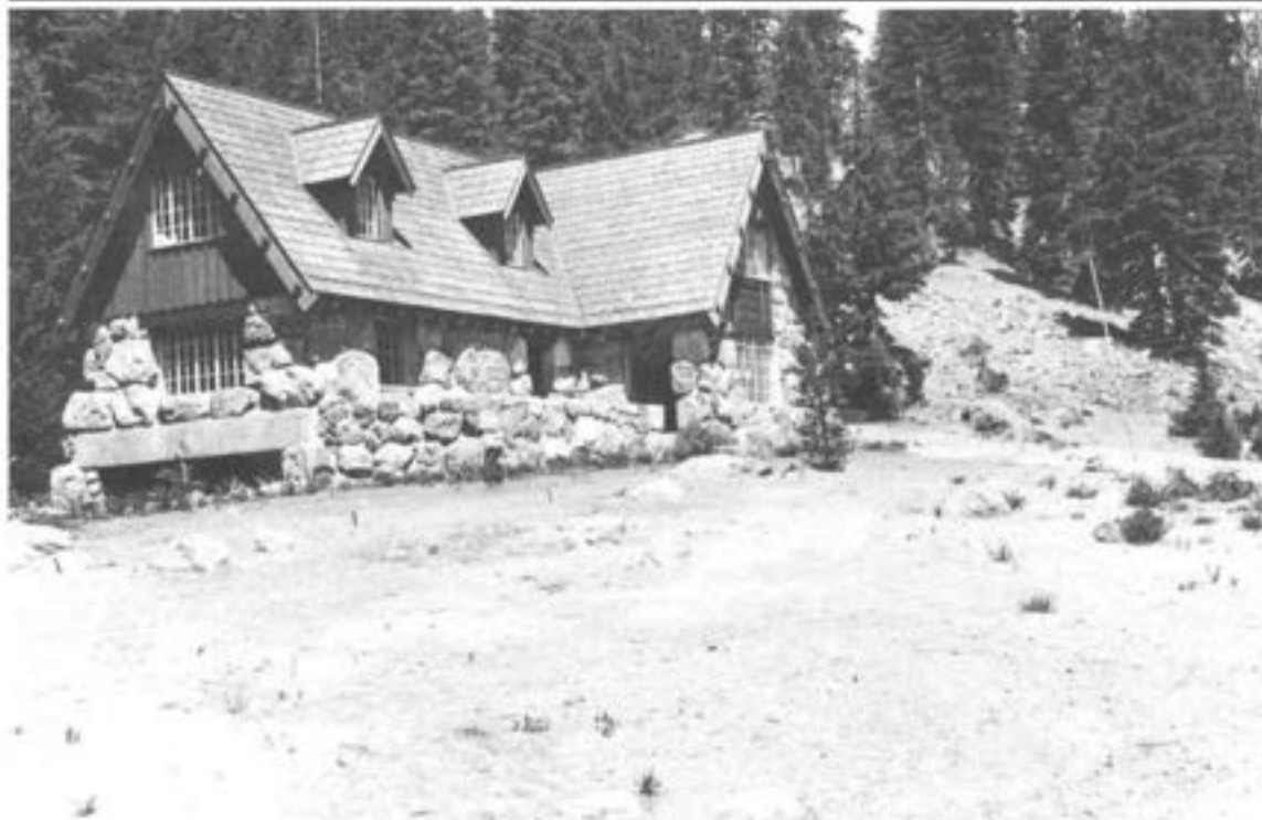
Historic photograph from 1934 of the Superintendent's Residence, prior to laying the flagstone walkway. Note the stakes near the building that outline the walkway. (CRLA/2637, 1934.)
