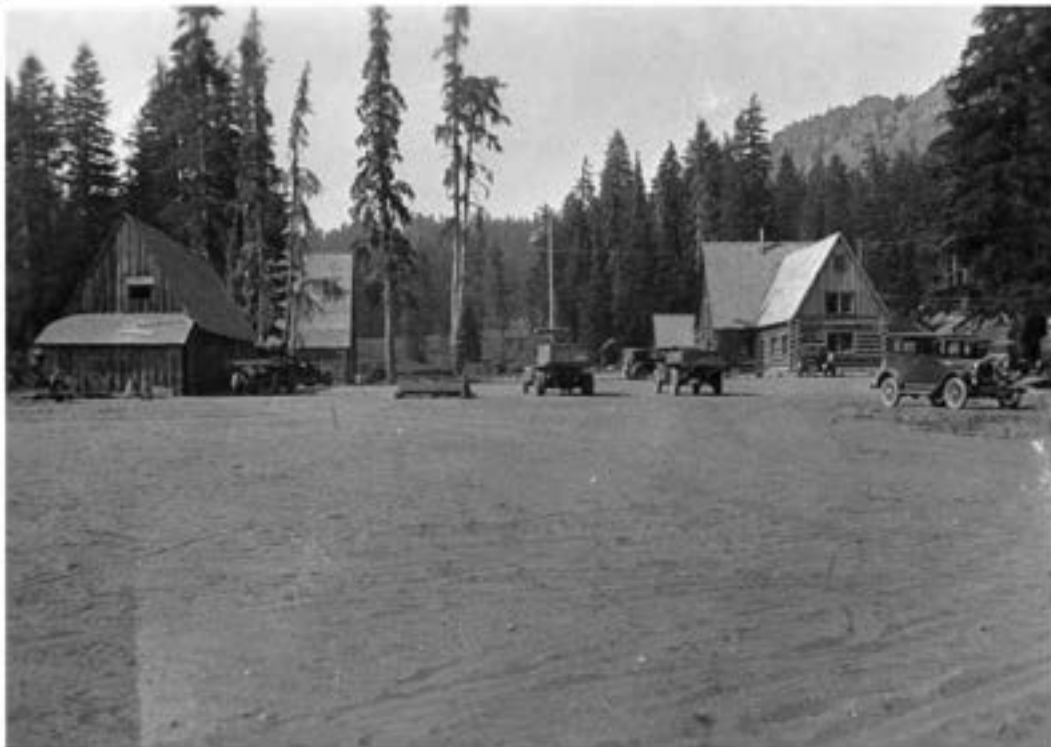
Historic photograph showing the early Park Headquarters at Munson Valley. (CRLA 206H 4268, ca. 1930.)
