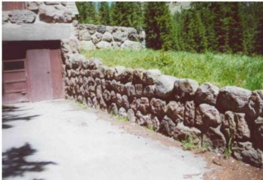
Contemporary photograph of one of the two rock and mortar walls that line the driveway to the garage of the Superintendent's Residence. (CCSO, 2000.)
