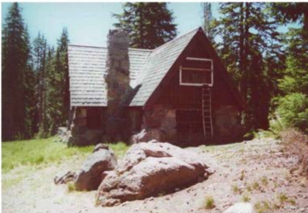
Contemporary photograph of the side façade (north elevation) of the Superintendent's Residence. Notice the large boulders in the foreground, that serve to blend the landscaped "yard" with the surrounding rugged terrain. (CCSO, 2000.)
