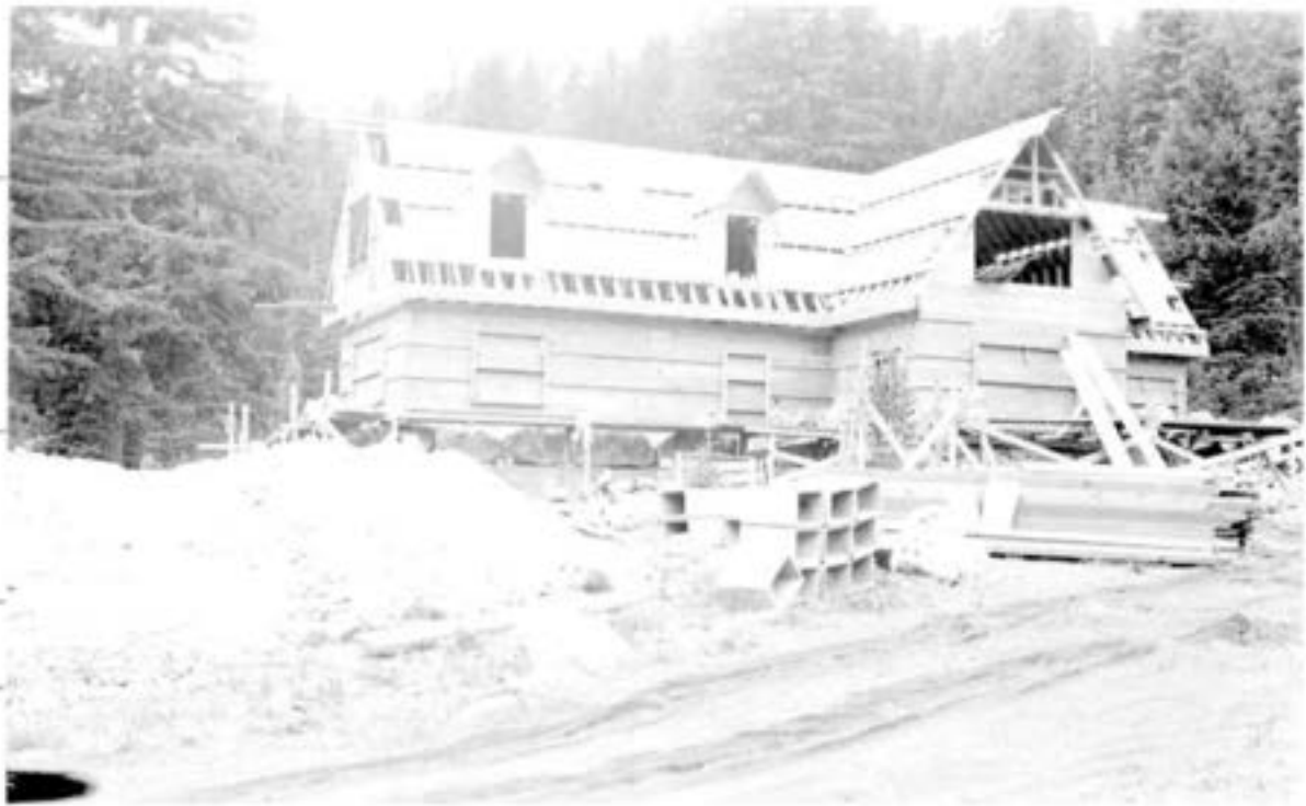
Historic photograph of the construction of the Superintendent's Residence at Munson Valley in 1932. Note the stonework being completed at the foundation of the building, and the crated coniferous tree at the front of the building. (CRLA/4363, 1932.)
