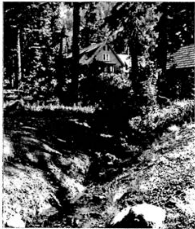
Munson Creek north of the Messhall in the administration area.
