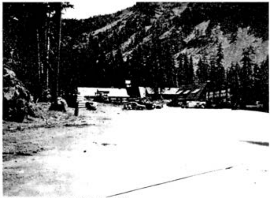
Maintenance area, looking north, 1990
