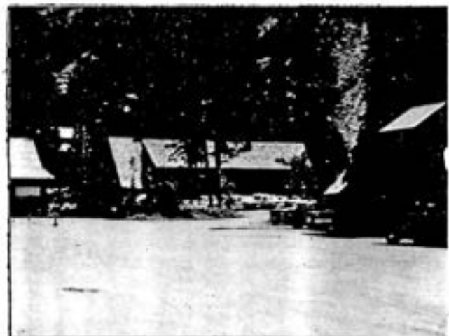
Maintenance area looking north. From left to right are the Warehouses, the current Ranger offices (Messhall), and Machine shop.
