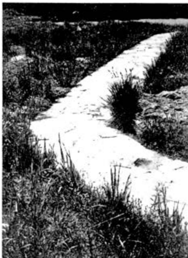
Flagstone walkway, Superintendent's Residence, west entrance.
