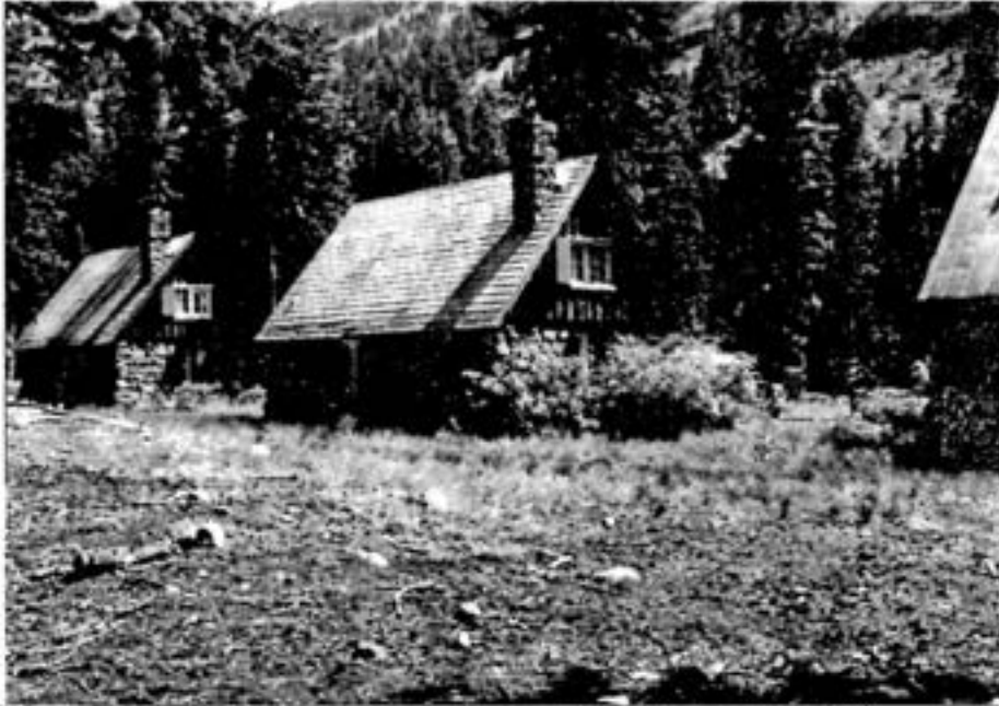
Lower group of employee residences on the spur road, rear view, 1990
