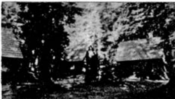
Sleepy Hollow cabins, c.1930 (cabins removed in 1989).
