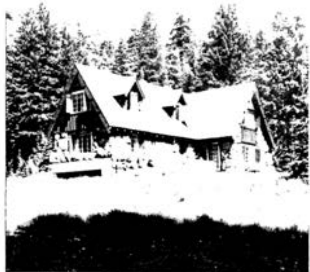
Superintendent's Residence, southeast view.
