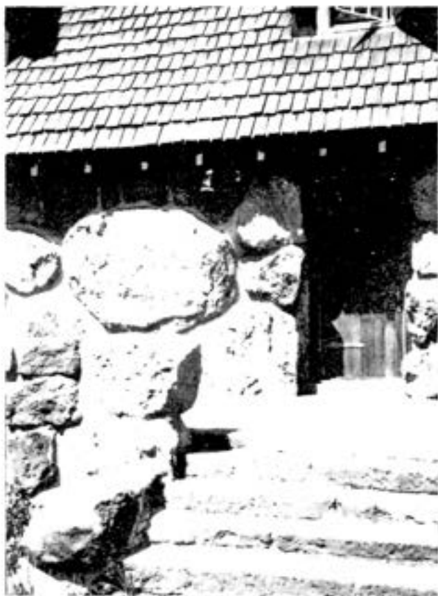
Superintendent's Residence, east entrance.
