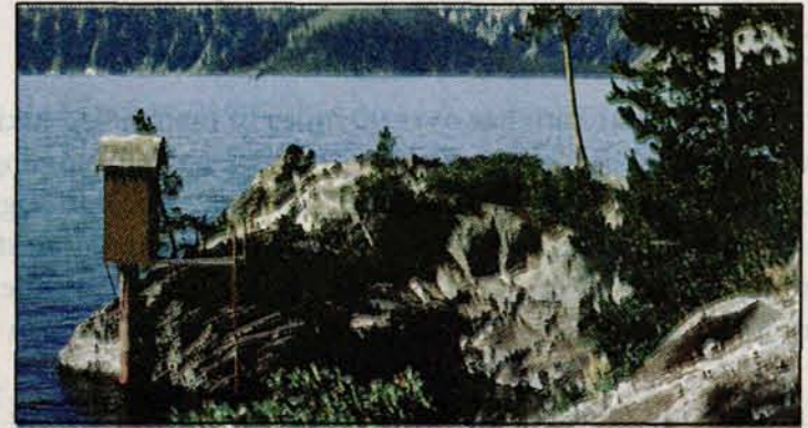
Lake surface level gauging station at Cleetwood Cove.
