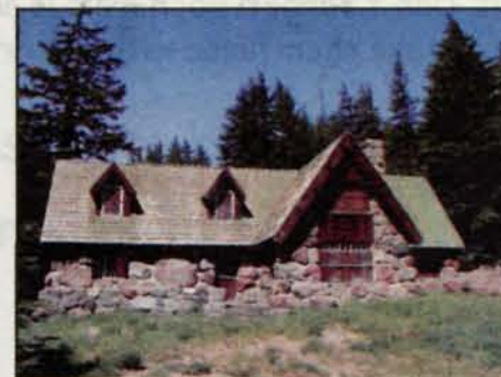
The historic superintendent's residence may house part of the proposed Science and Learning Center
