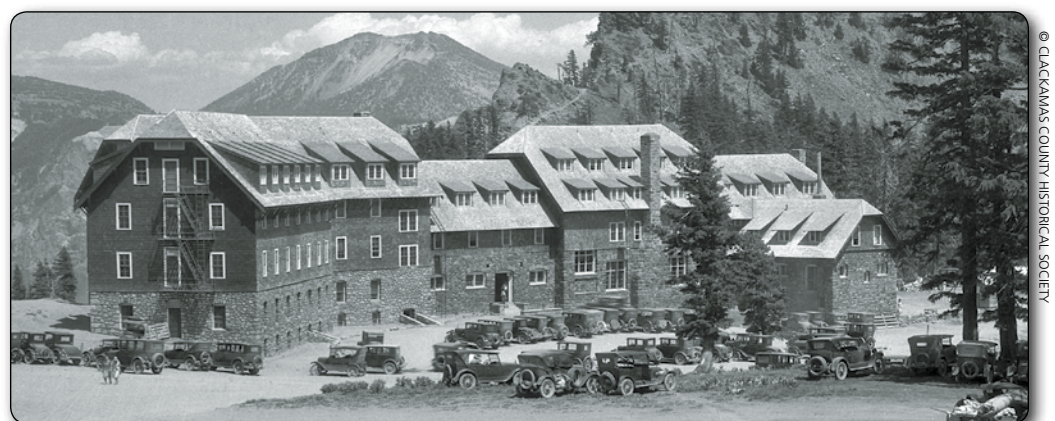
The original lodge was a wood frame atop a rock wall. Its stones were quarried from Garfield Peak and Watchman Peak. It achieved its present-day form in the 1920s, with the addition of two wings of rooms on the west side of the building. When it was rebuilt in the 1990s, architects preserved its external appearance but transformed the interior into a modern—and structurally sound—facility.
