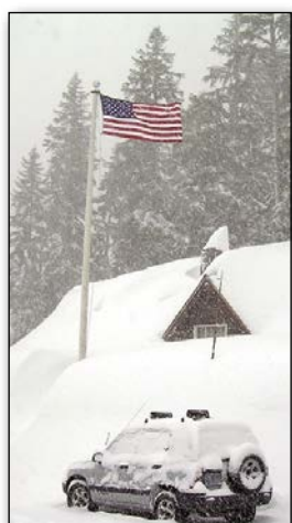
Steel Visitor Center
