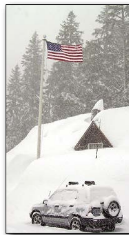
Steel Visitor Center
