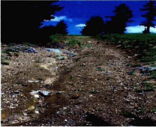
Soil erosion on the old Lodge Dump Road.
