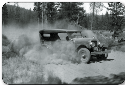
Until the 1930s, when park roads were paved, deep sand and choking dust frustrated motorists.
