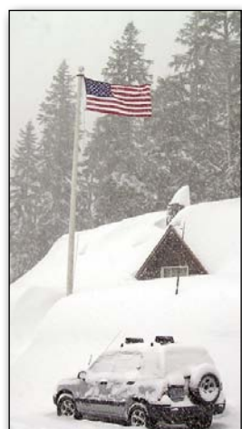
Steel Visitor Center
