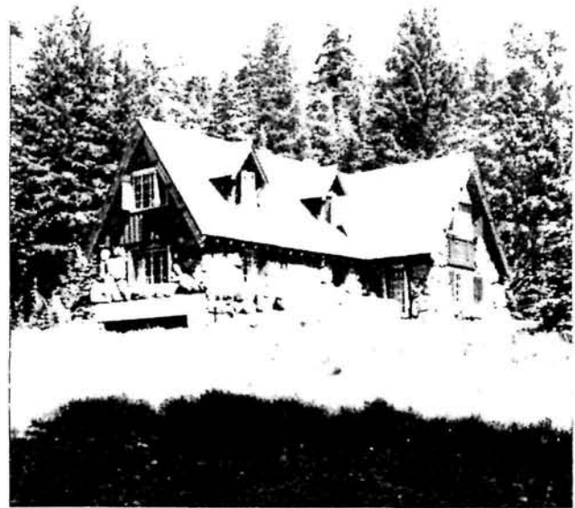
Superintendent's Residence, southeast view.
