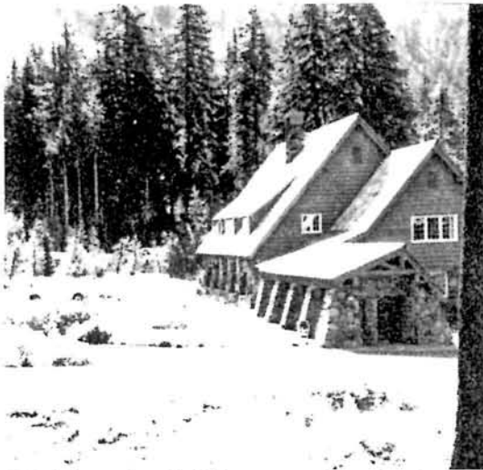
Administration Building; west view showing the snow tunnel and north parking lot.
