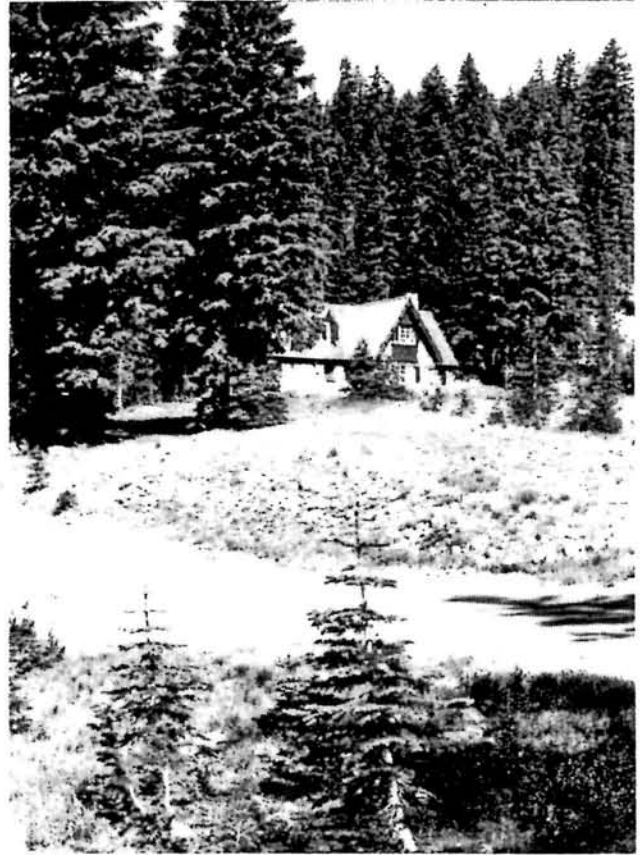
Access road and meadow at Superintendent's Residence, looking northwest.
