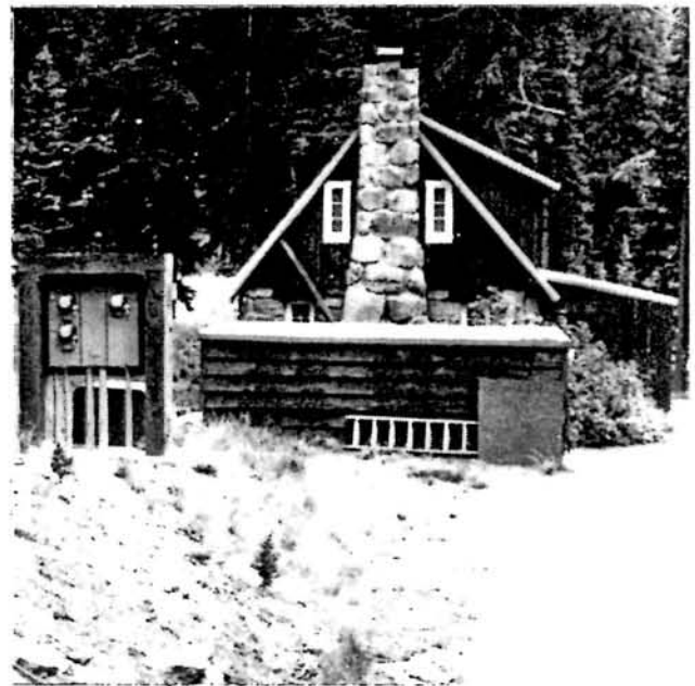
Utility box at the middle group of employee residences.
