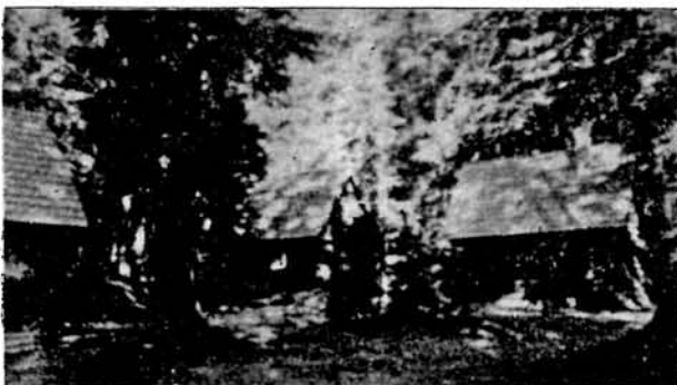
Sleepy Hollow cabins, c.1930 (cabins removed in 1989).
