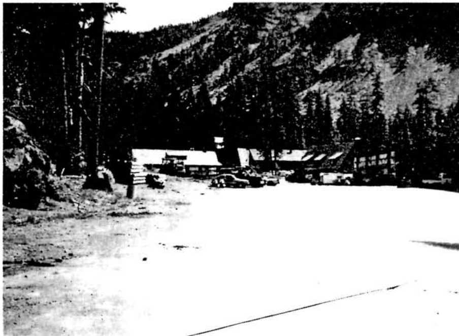
Maintenance area, looking north, 1990
