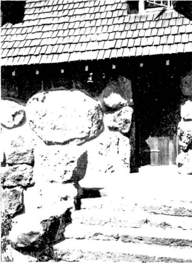
Superintendent's Residence, east entrance.
