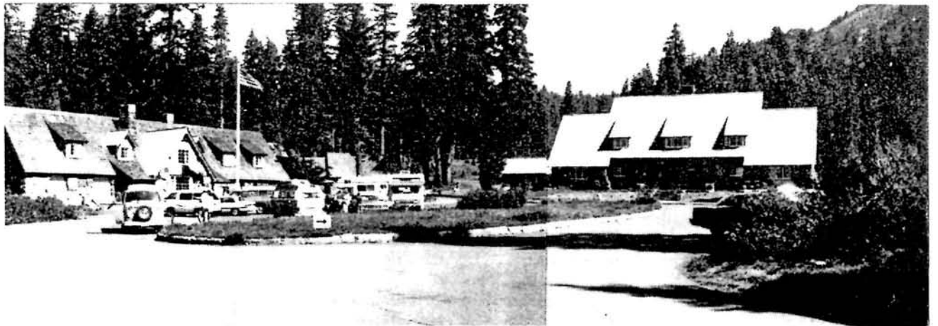
Administrative plaza looking north from the entrance; Ranger Dormitory (left), Administration Building (right).
